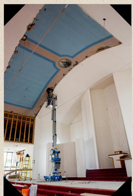
The old ceiling tiles have been removed and the celestial ceiling is being prepared.
